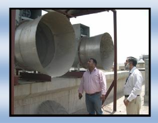
Renowned Consultant Fahim, Nanji & DeSouza & Co, initiated enquiry for high performance ventilating fans for their project at Sapphire Finishing Mills Ltd in Raiwind with very high specs. Tube Axial Inline Fans based on 50C ambient temp., with chemical resistance coating to avoid rust / damage for longer life as previously used fans lasted only in 1-2 years.
