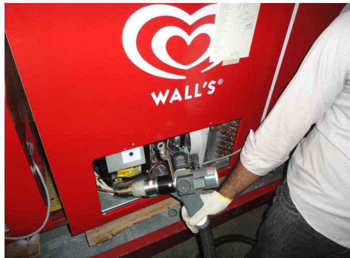
REFRIGERANT R290a CHARGING in SECOP COMPRESSOR
