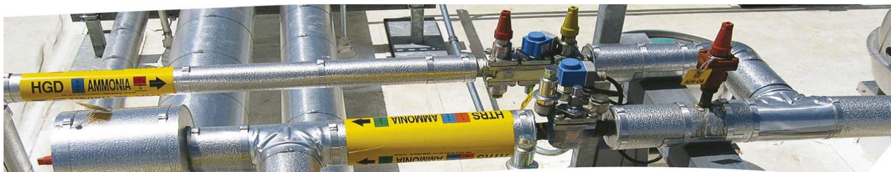
Fig 3: Danfoss Ammonia Control equipment.
